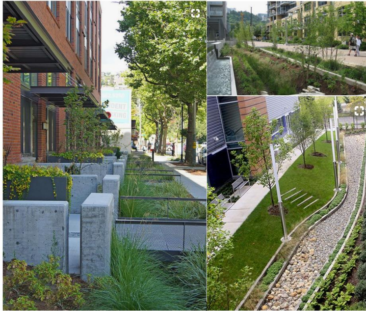
Figure 5-1: Examples of Urban Swales/Bio-swales – Various Sources
